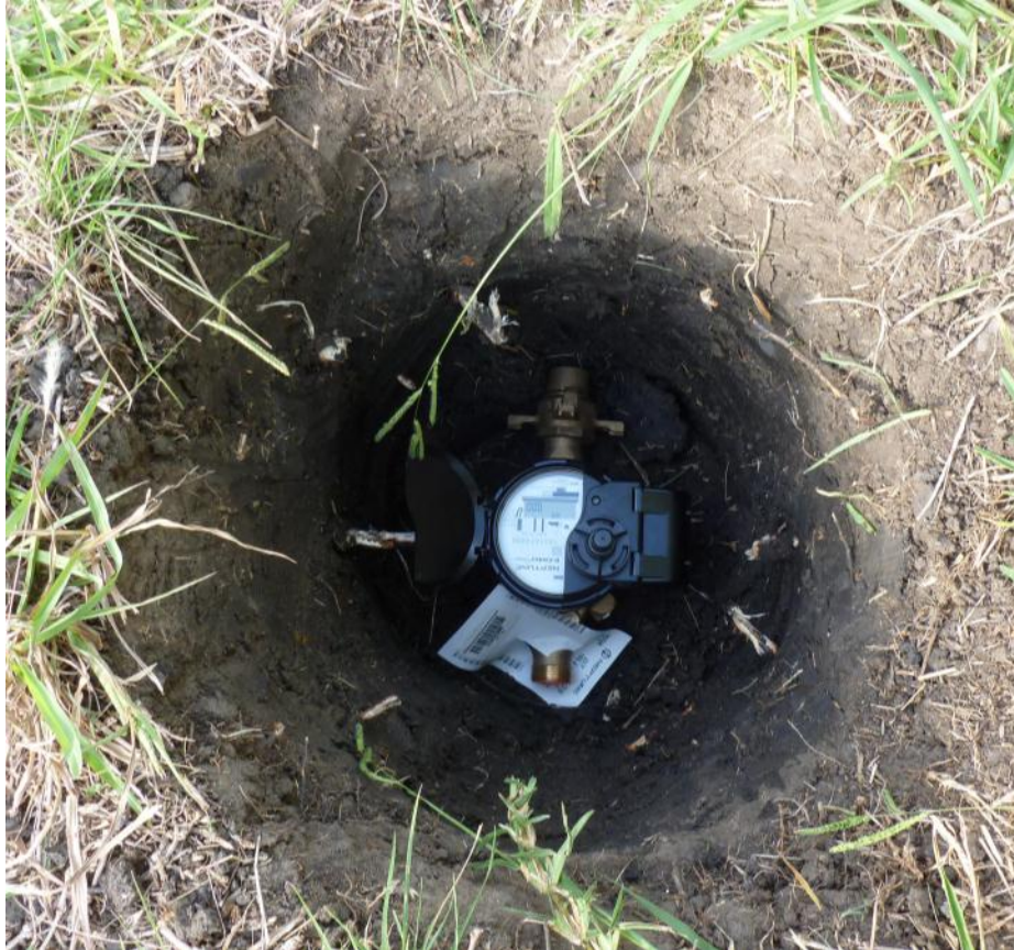
The Neptune water meter located inside a hole in the ground, as it would be placed by the water company. The antenna is the small round bulge on the top of the right side of the meter body.
